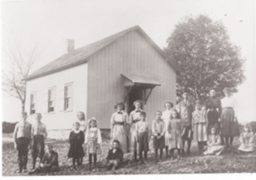
The Long Ridge School, one of our 1-room schoolhouses
